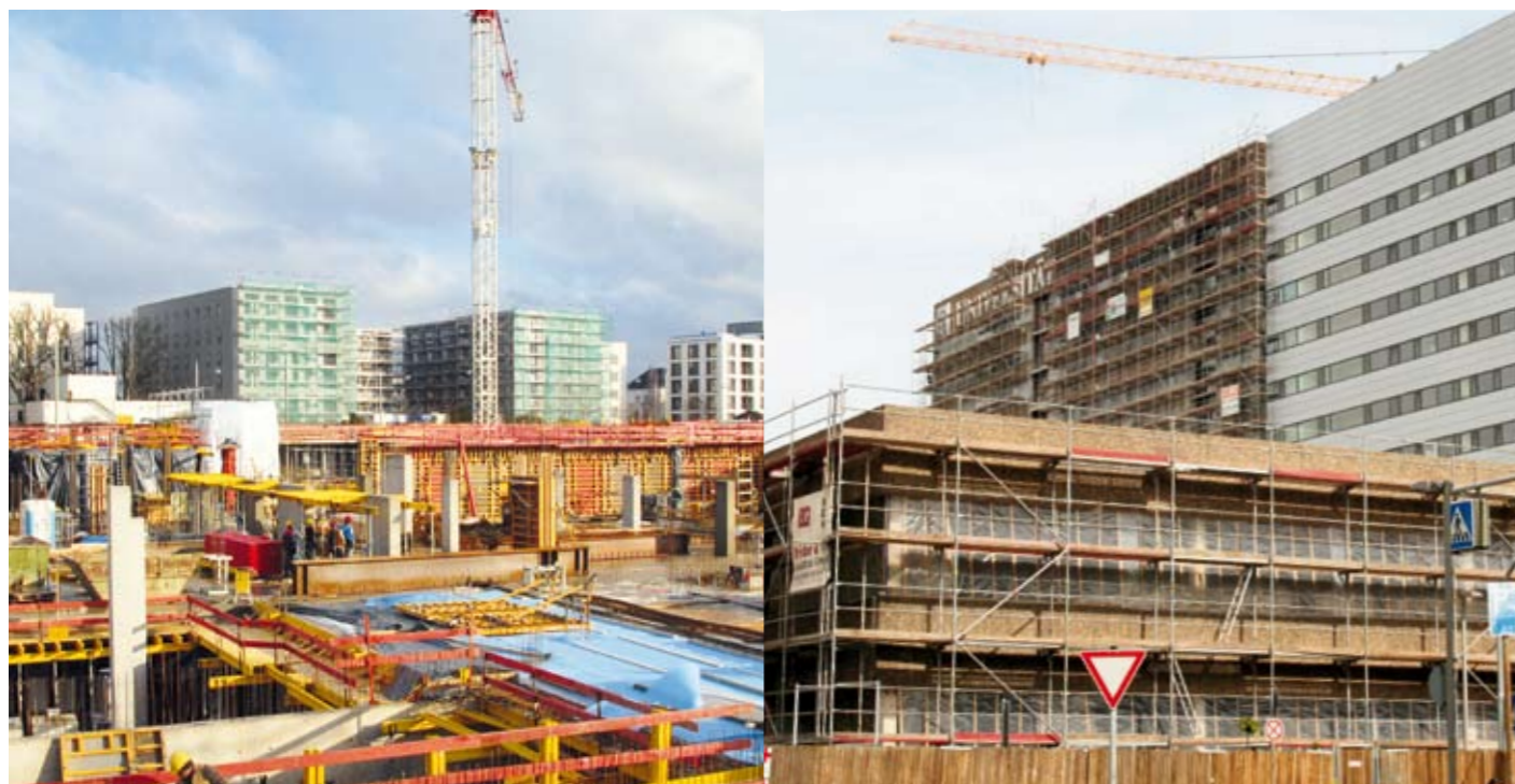
Massive construction works at the Campus Westend (left) and Universitätsklinikum.
